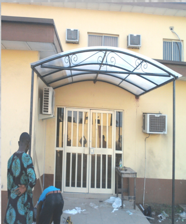
Entrance Canopy Installation
