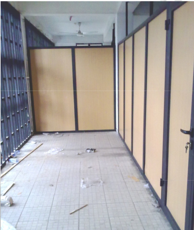
Office Partitioning for Octagon
