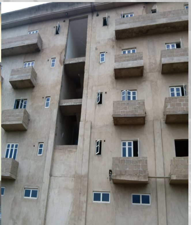
Aluminium Windows Installation
